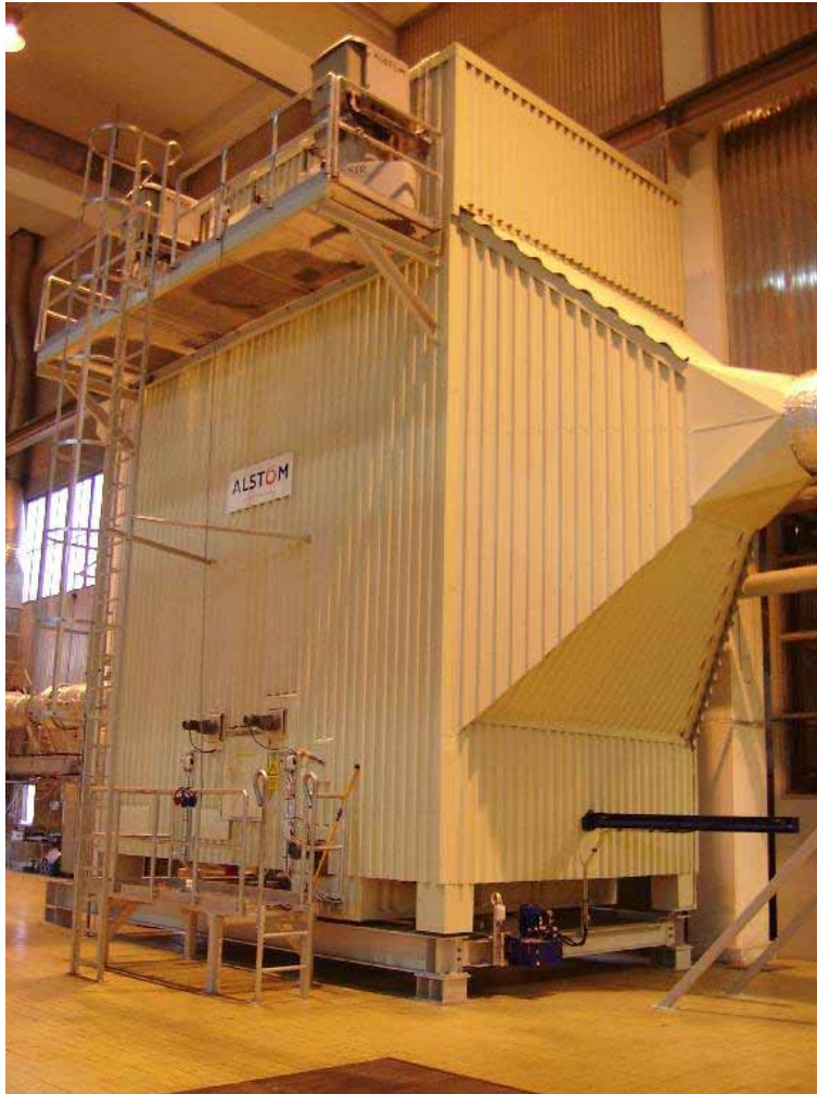
External view (inlet of ESP)
